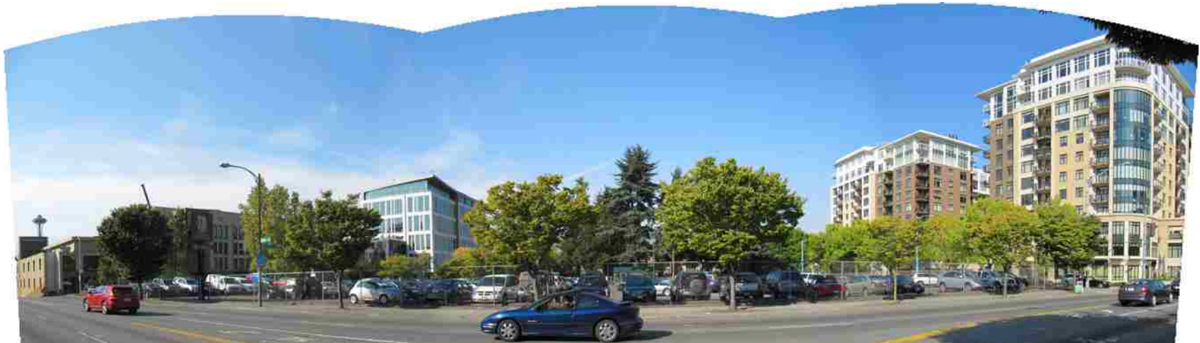
Figure 6.7 Existing site conditions.
